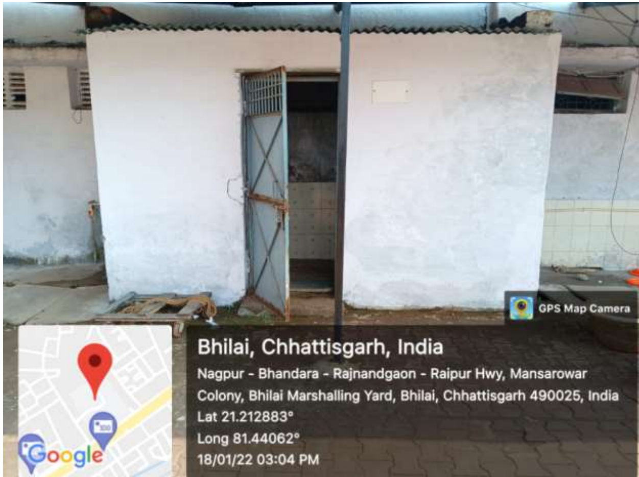
Girl's Toilet in Old Building
