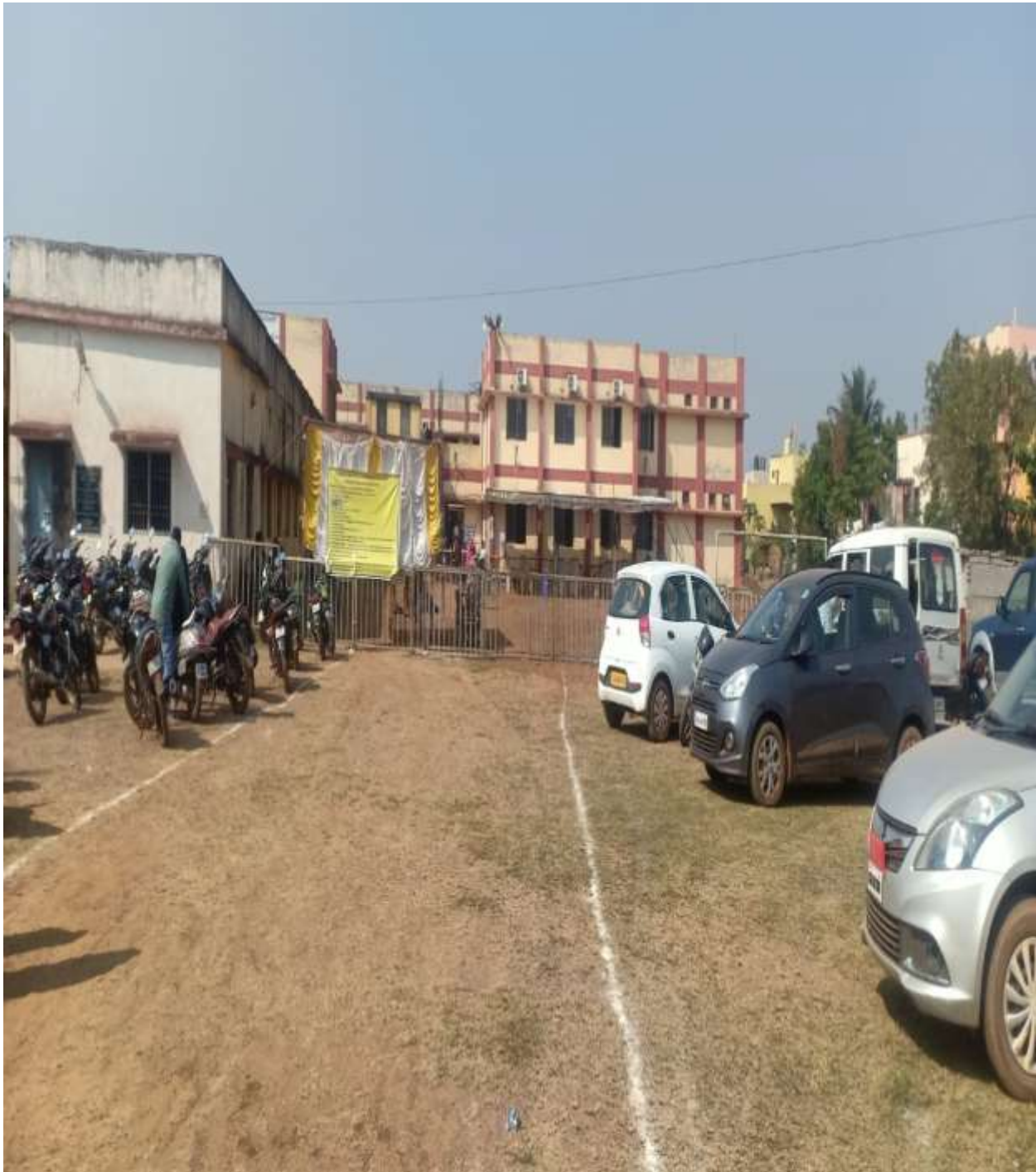
College New Building
